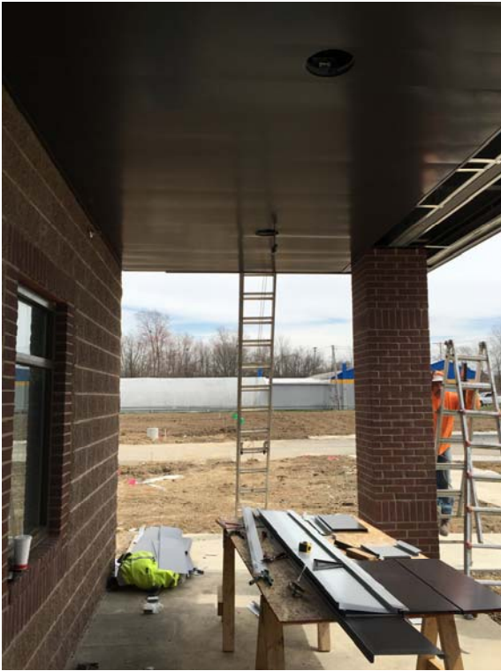
Brick columns and canopy with metal soffit panels. Storefront entry installed at vestibule and in lobby.
