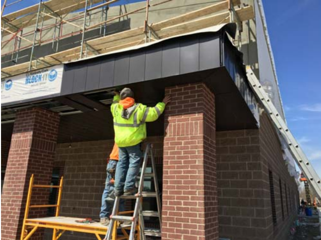
Views of canopy metal fascia and soffit panels.
