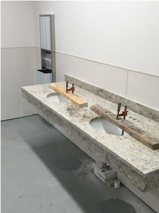
Granite countertop and backsplash installed. Paper towel dispenser & waster receptacle installed. Urinal installed, toilets have yet to be installed. Flush valves have not yet been installed. Restroom wall and floor finish installed. Grab bars have been installed.
