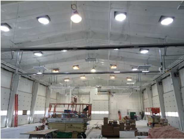
Views of the garage with the solartubes installed. Radiant heaters have been installed. Interior painting have been completed. All utility lines have been installed.
