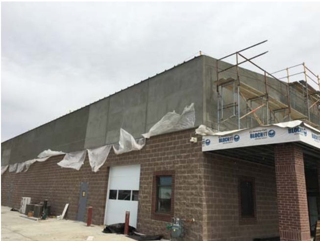
Installation of EIFS with control joints and reveal
